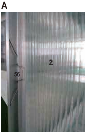
photo of fixing the 4mm roof panel
