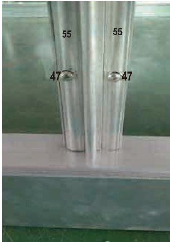
photo of fixing the clear wall panel
