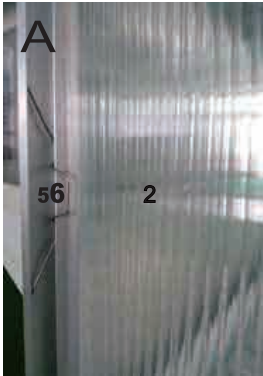
Using number 56 clip to fix the roof panel
