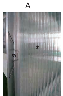
photo of fixing the 4mm roof panel
