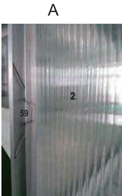
photo of fixing the 4mm roof panel
