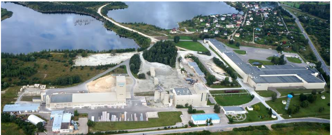
KNAUF Sauriesi, Stopinu novads production plant in Latvia
