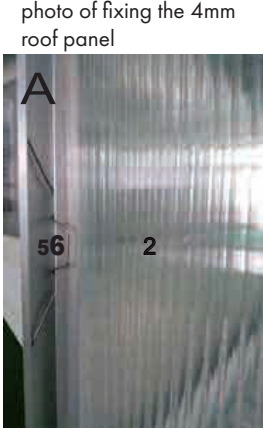
Using number 56 clip to fix the roof panel
