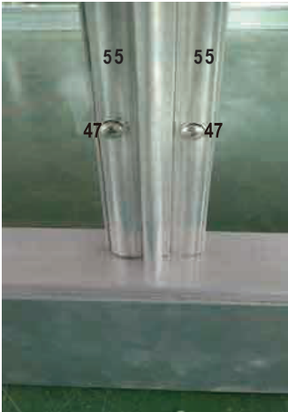
photo of fixing the clear wall panel
