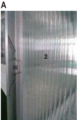
photo of fixing the 4mm roof panel
