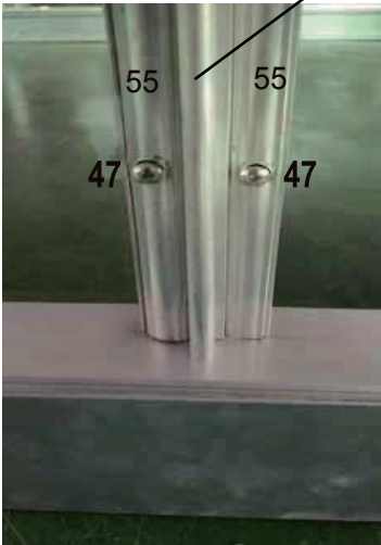
photo of fixing the clear wall panel
